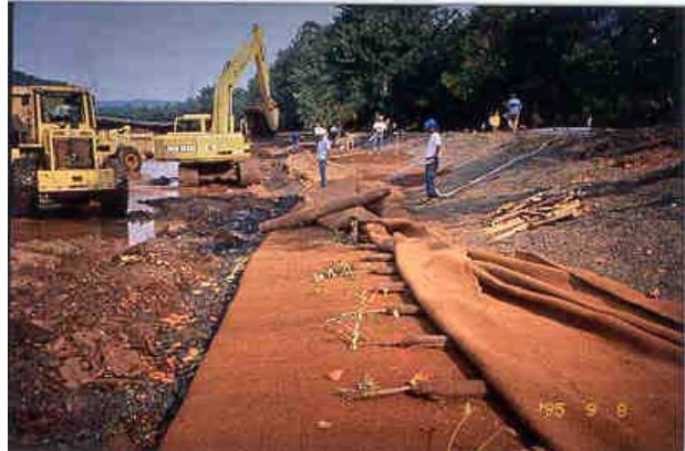
Raritan River During Construction
